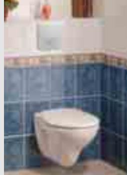
Tank recessing allows the creation of a shelf. Toilet will become more modern.
